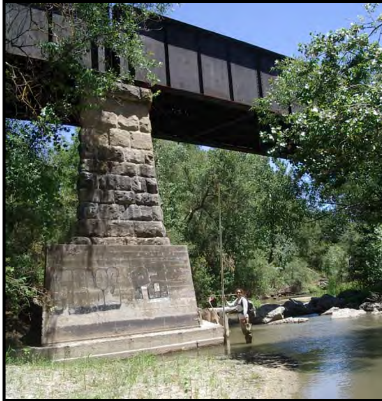
Figure 79. Photograph (looking downstream) showing that the bed level is currently approximately 3 m below the stone portion of the abutment for the upper railroad bridge (formerly Southern Pacific, now owned by Union Pacific). Stadia rod is 5 m in total.
