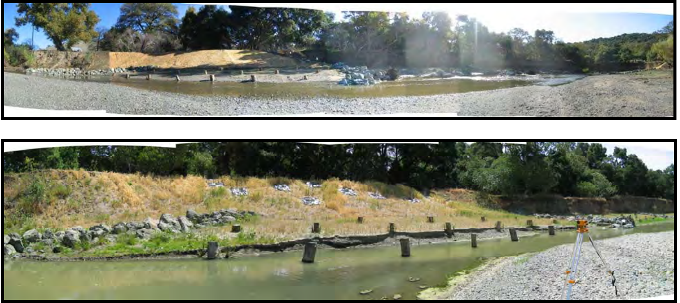
Figure 72. Panoramic photos showing bank stabilization project in upper subreach of Arroyo De La Laguna (top photo from November 2006, bottom photo from May 2007). Flow is from left to right.
